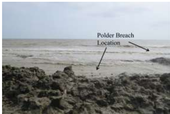
Fig. 3: Breached sea-facing polder at different locations of Banshkhali Upazila.
